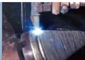
Build-up welding of an axial roller with UTP AF DUR 550 MP
